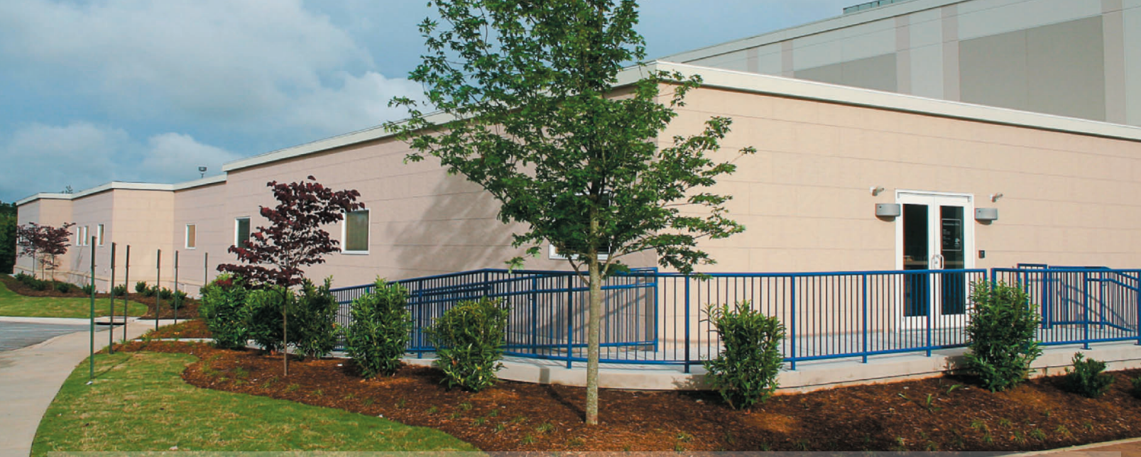
SIDE BACK VIEW OF THE BUILDING ORPE CHARITY CLINIC PROTOTYPE - 12,000 square feet
