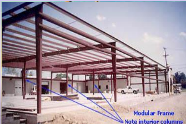
STEP 5: Prefabricated structure (with 50 year warranty) will be installed to the building foundation to give the building an architectural of awesome appearance. The siding material may be applied directly on top of the concrete slab.
