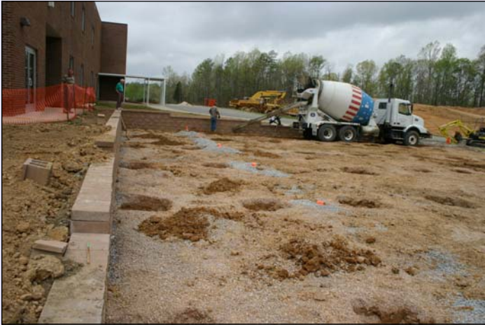
STEP 1: The site is prepared with a concrete retaining wall and poured concrete footings at the same time the building is being prefabricated by the manufacturer.
